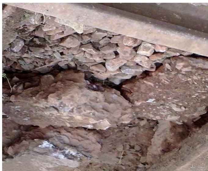
Figure 3: The local effects of excessive clogging ( >> 30\% ) of the crushed stone prism- the emergence of very harsh portions (conglomerates).
